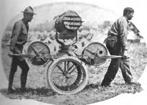
Searchlight apparatus on Autocar truck which can be hauled ½ mile away from source of current
